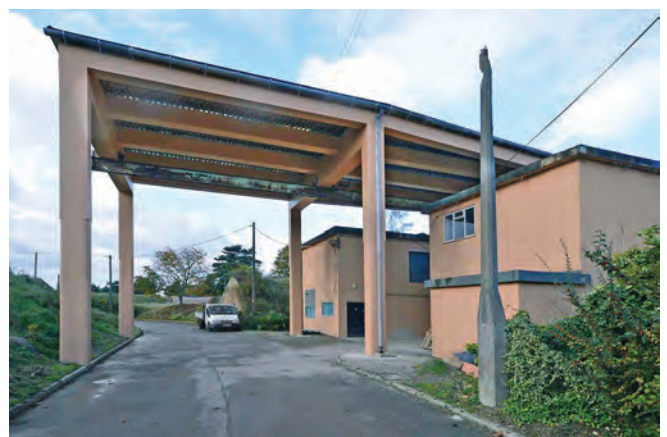
Side view of Non-nuclear Component Building 60's gantry, which was required to lift and manoeuvre the massive Blue Danube bomb onto a bomb trolley for wheeling into the building
